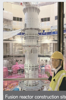
Fusion reactor construction site
